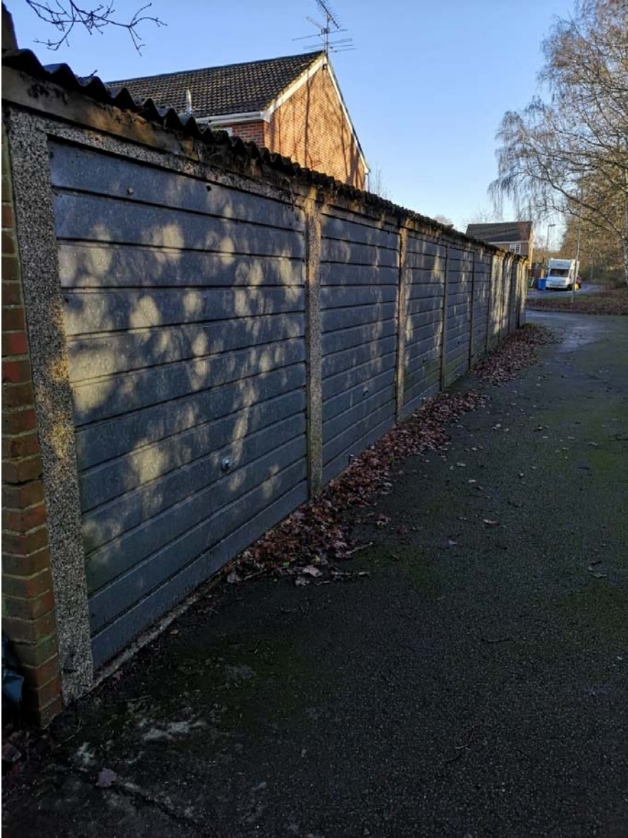
Photograph 7.7.1: Stakes Lane garages, 16/01/2019, standard lens
