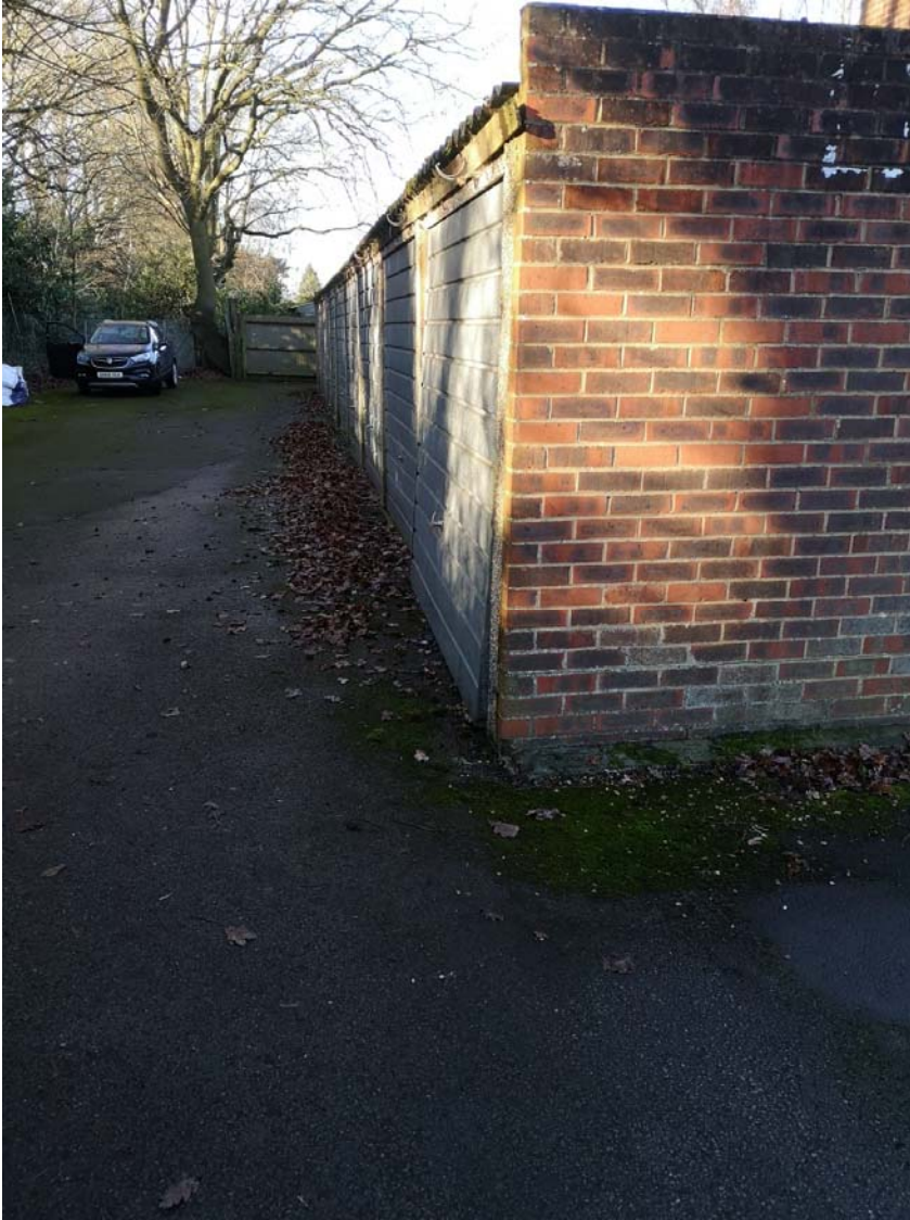
Photograph 7.7.3: Stakes Lane garages, 16/01/2019, standard lens
