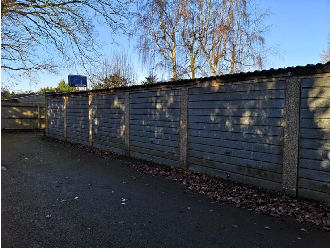
Photograph 7.7.2: Stakes Lane garages, 16/01/2019, standard lens
